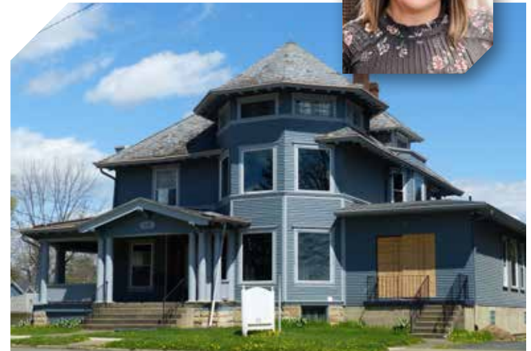
New Directions' new facility in process of renovation.
